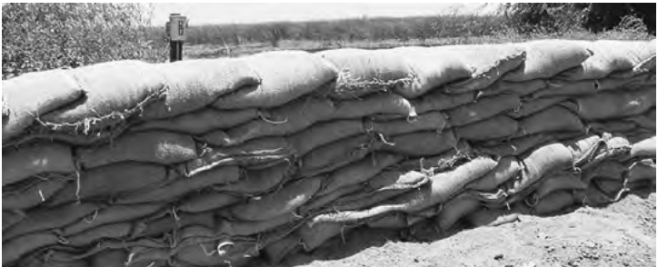
Sandbag Wall Construction
